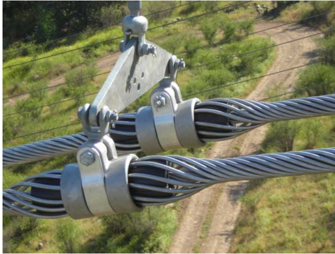
Picture of PLP suspension AGS system.
